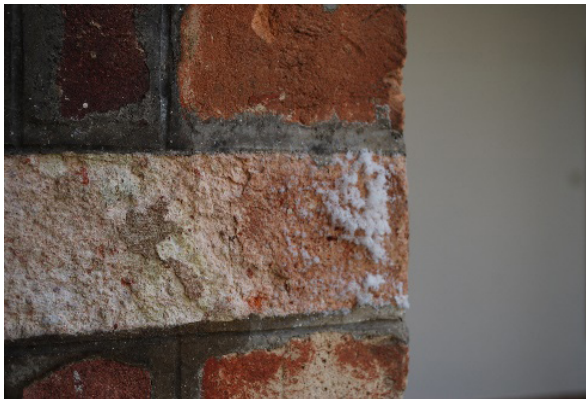
Photo 10: The effect of salting or efflorescence on wall surfaces Source: Sultan Abdul Samad Building Façade Conservation Project, 2009
