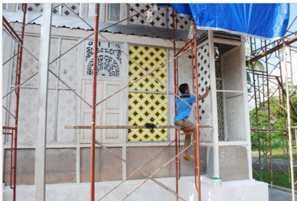
Photo 20: Painting work on the 'kelarai' woven bamboo wall Source: Ihsaniah Iskandariah Mosque Conservation Project, Kampung Kuala Dal, Perak, 2015
