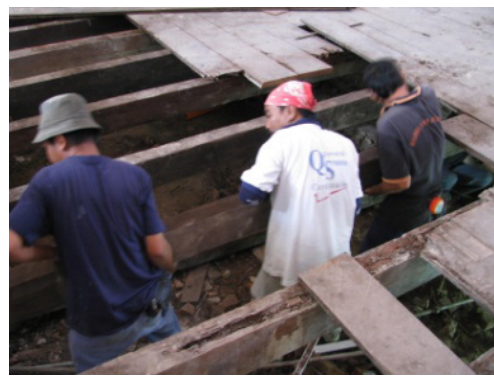
Photo 12: The main damage to the floor is wood rot which is due to dampness and termite attack. Left and right photos are works on removing damaged floor joists and floor boards Source: Taiping Museum Conservation Project, Perak, 2008
