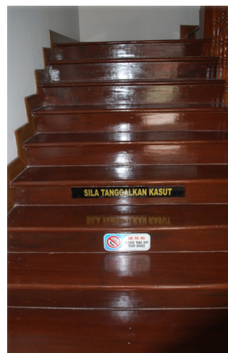
Figure 22: The wooden staircase in a heritage building portrays unique construction and is usually made of local hardwood species
