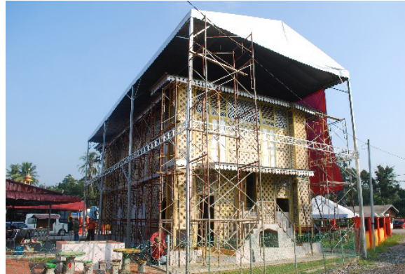
Photo 3: Temporary roof needs to be constructed before any conservation works commence Source: Masjid Ihsaniah Iskandariah Conservation Project, 2015
