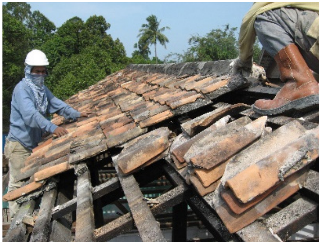
Photo 5: Disassembling the roof tiles for cleaning works
