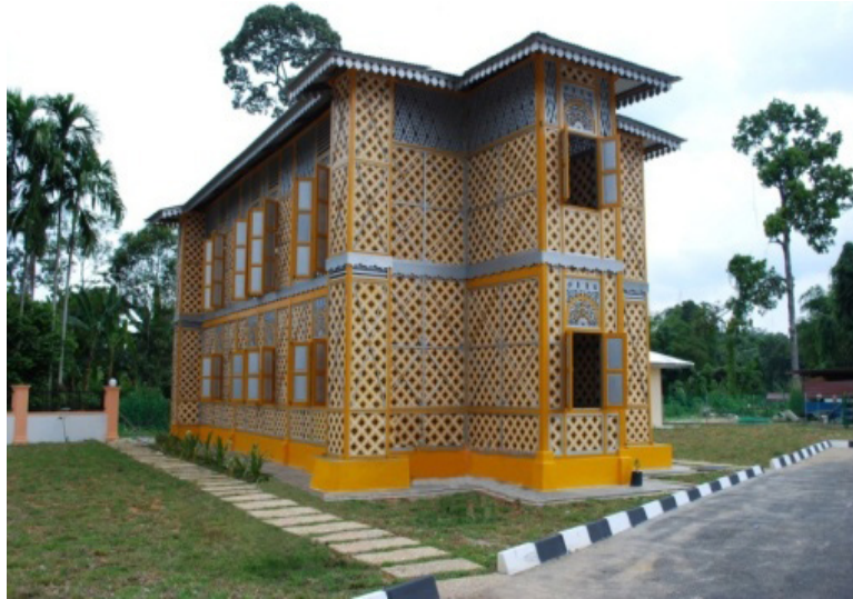
Photo 1: Ihsaniah Iskandariah Mosque, Kampung Kuala Dal, Kuala Kangsar, Perak is a building made of kelarai or woven bamboo strips constructed in 1938.
