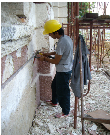
Photo 7: Brick replacement and repairing of damaged plaster Source: HSBC Building Conservation Project, Melaka, 2009
