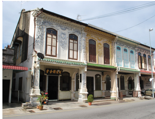
Photo 18: A row of shophouses displaying unique decorative mouldings on the façade, Kampung Cina, Melaka
