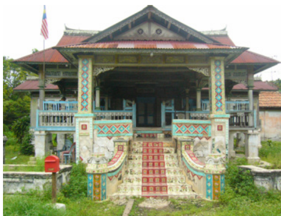
Photo 21: The stone staircase at the Penghulu Natar House, Melaka. The staircase of this 'rumah ibu' or main house section has an attractive traditional staircase with patterned tile finishes Source: Penghulu Natar House Conservation Project, Melaka, 2009
