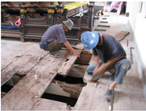
Photo 12: The main damage to the floor is wood rot which is due to dampness and termite attack. Left and right photos are works on removing damaged floor joists and floor boards Source: Taiping Museum Conservation Project, Perak, 2008
