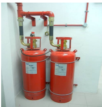
Photo 23: Dry Powder Fire Prevention System Installation Source: Conservation Division, 2015
